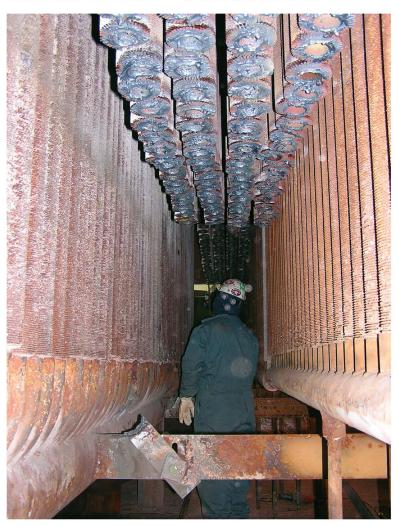
A power producer with a **Nooter/** Eriksen HRSG which had been operating for over 10 years had experienced unacceptable backpressure levels in their unit over the past few years. The backpressure increase was caused by fouling of the finned tubes, primarily in the LP Economizer coils in the "cold" end of the HRSG. These coils in some operating cases fall below the dew point temperature of certain compounds that condense out of the exhaust gas. The fouling in this case had
